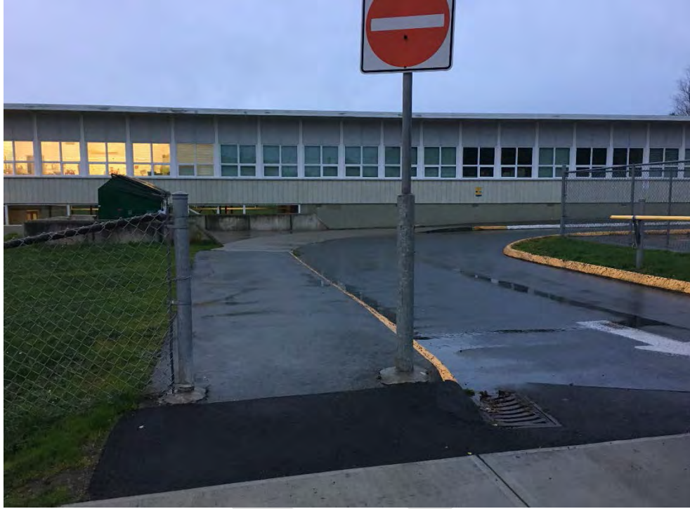
Figure 3 - Drop-off zone exit
