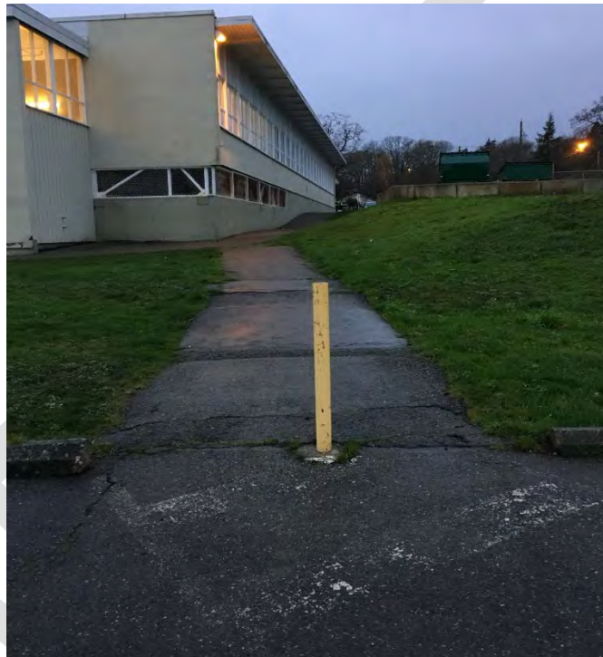
Figure 10 - First pedestrian path from staff parking lot to school grounds
